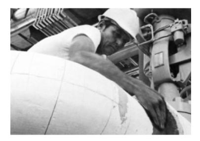
Materials' Marinite Insulating and Finishing Cements are air-setting materials, mixed with water and applied in plastic form. They are designed for application to irregular surfaces where it is impractical to cut and apply pipe, block or other insulating products.
