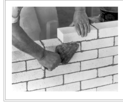
R efractory Bonding Mortars are finely ground refractory materials which are plastic, or become plastic and trowelable when mixed with water. Our mortars are suitable for laying and bonding insulating fire brick and most clay-based dense fire brick.
